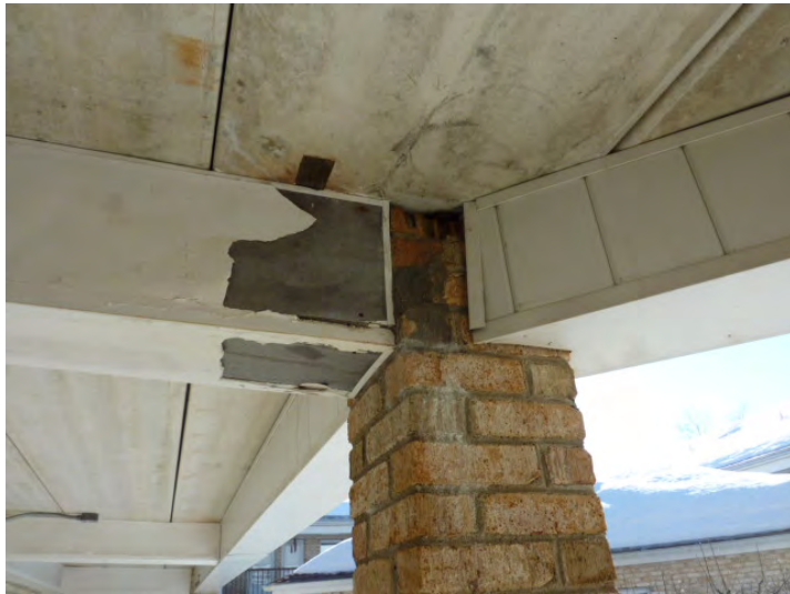
Rusting steel plates and cracked brick joints are signs of typical ongoing distress at the column beam connections.
