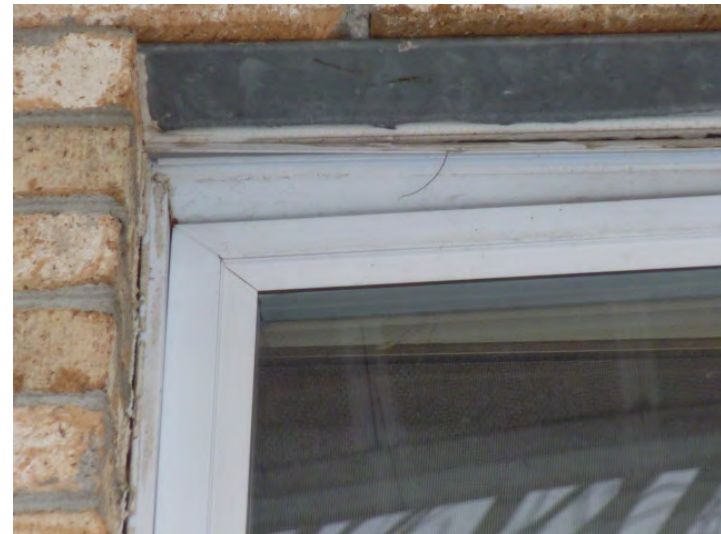
Windows are the originals and are 24 years old. Worn finishes, failing caulking and sash misalignment are all typical.
