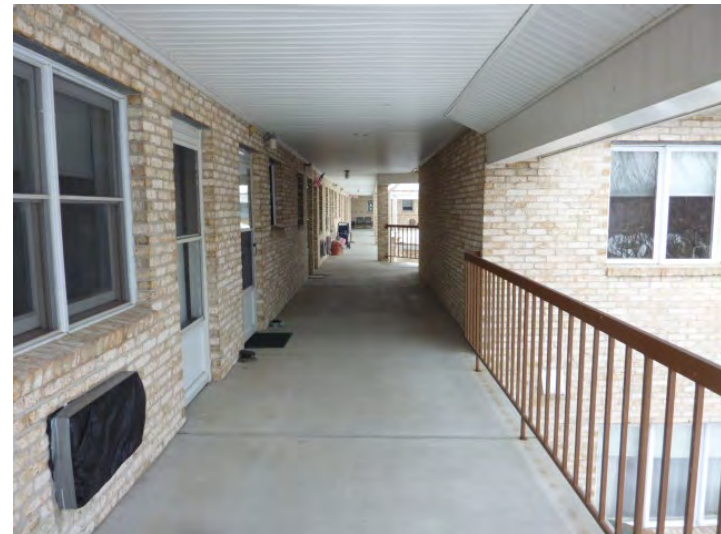
Typical single loaded second floor walkway with typical abandoned air conditioner sleeve.
