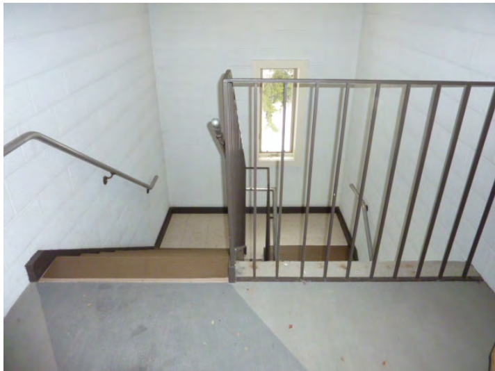
Typical stair with handrails, not the required guardrails at landings; handrail should also be continuous on all walls.
