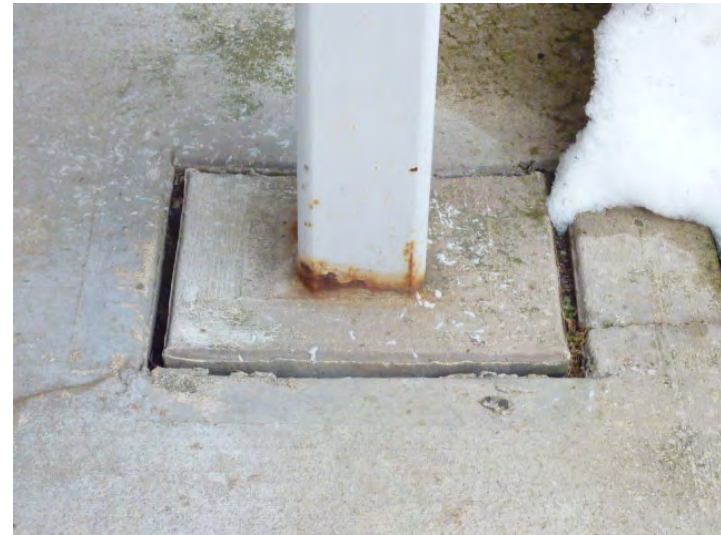
Typical rusting at column base where it is unprotected from moisture.
