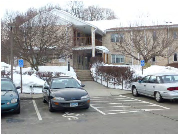
Asphalt walks at the main entrance at the southwest corner of the courtyard and site-wide are in poor condition.
