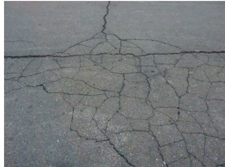
Typical asphalt driveway paving sub-base failure.
