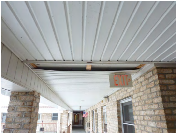
Typical vinyl soffit failure.
